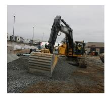
"Being able to set grade in aggregate for our pipe has been a huge difference," he said. "In Auto mode, my operator can get a perfect grade every time, so the gravel savings is substantial. We've found that we can save about 10 tons of material on a 100-meter stretch. At today's prices for aggregate, those savings can be substantial."
