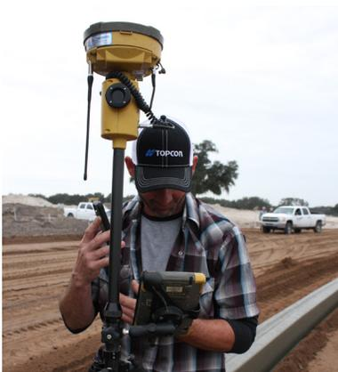
no way it could do that using just GPS," he said. When he was shown how Topcon had combined it with laser technology to bring it to millimeter grade, he decided it was time to give it a serious look. "We added it on a Power Curber 5700C and were immediately impressed with what we were able to do."
